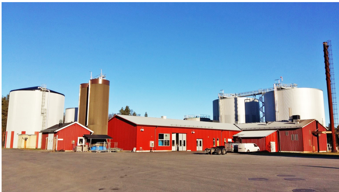
Biomar® wastewater treatment plant with 2 Biomar AWR-reactors (right) and a Biomar OSB-reactor (left)
